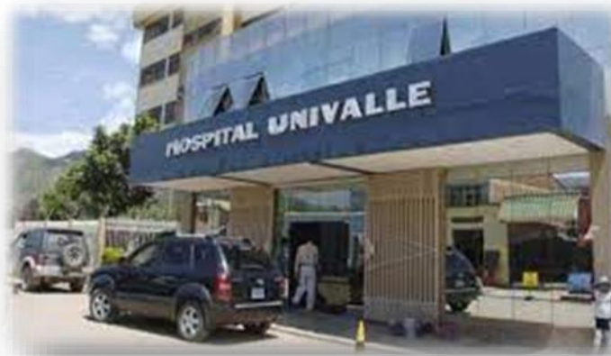
COCHABAMBA Hospital Univalle Sinfa S.A.
